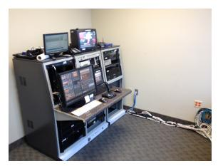
The equipment is now more organized and takes up less space. The racks are in 2 parts with the main part (left 2 racks) able to be serviced from both sides and the audio/presentation rack (right rack) able to pull fully out.
